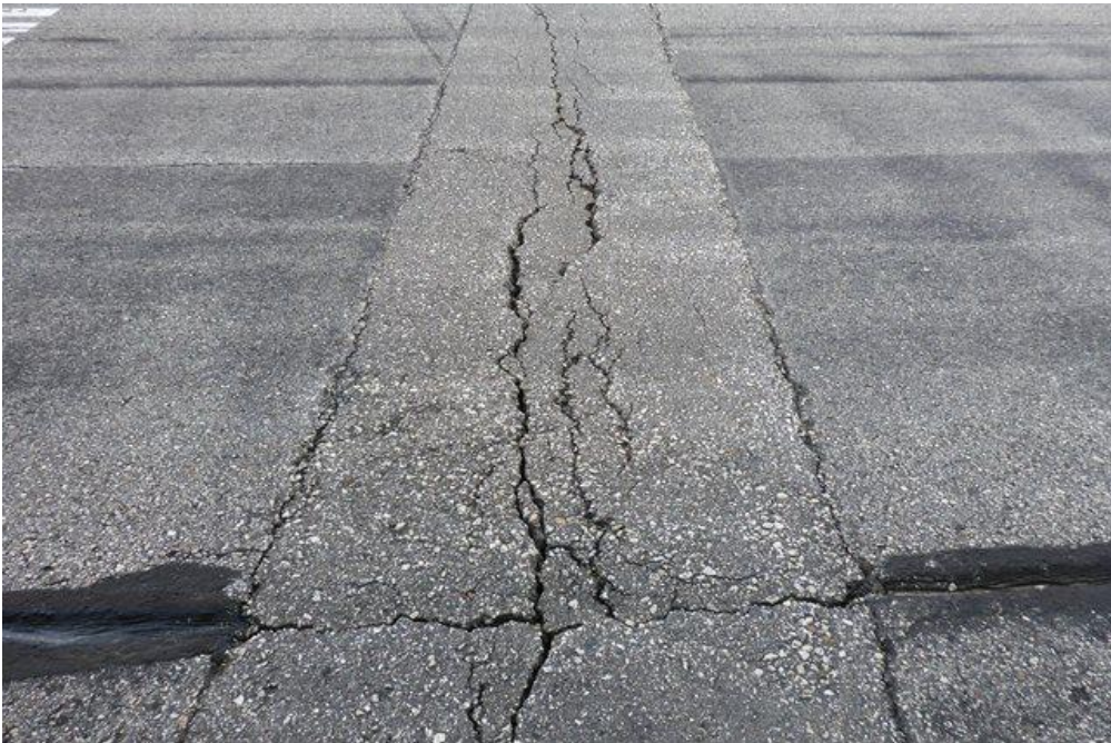
ONA RY1230 001 (Photo prior to 2015 Rehabilitation)
