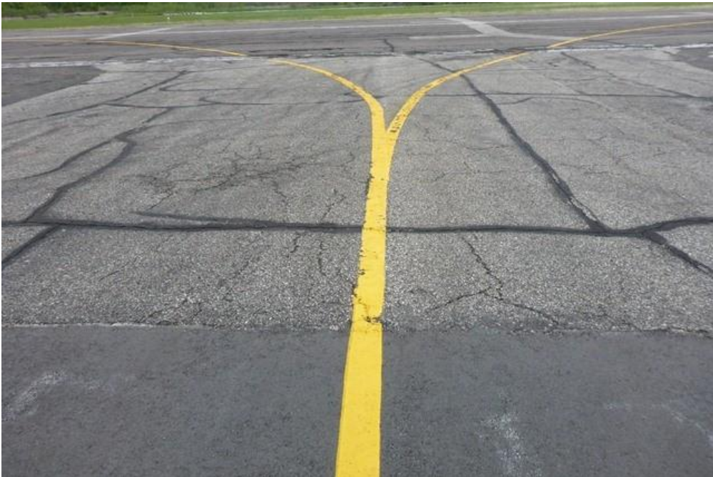
ONA CTA3 002 (Photo prior to 2015 Rehabilitation)
