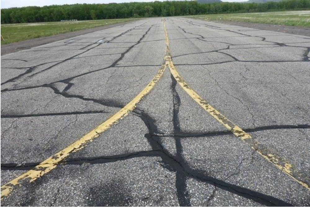
ONA CTA4 001 (Photo prior to 2015 Rehabilitation)
