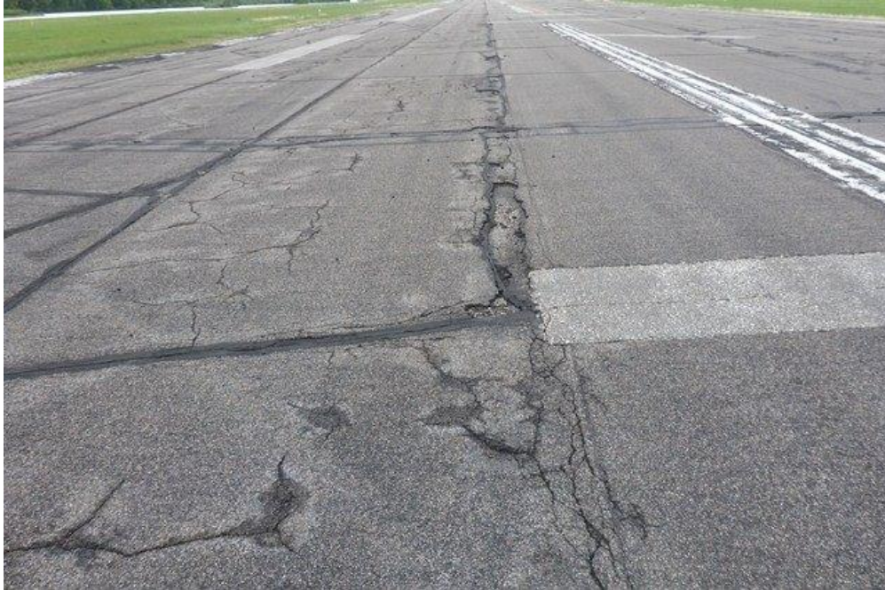
ONA RY1230 001 (Photo prior to 2015 Rehabilitation)
