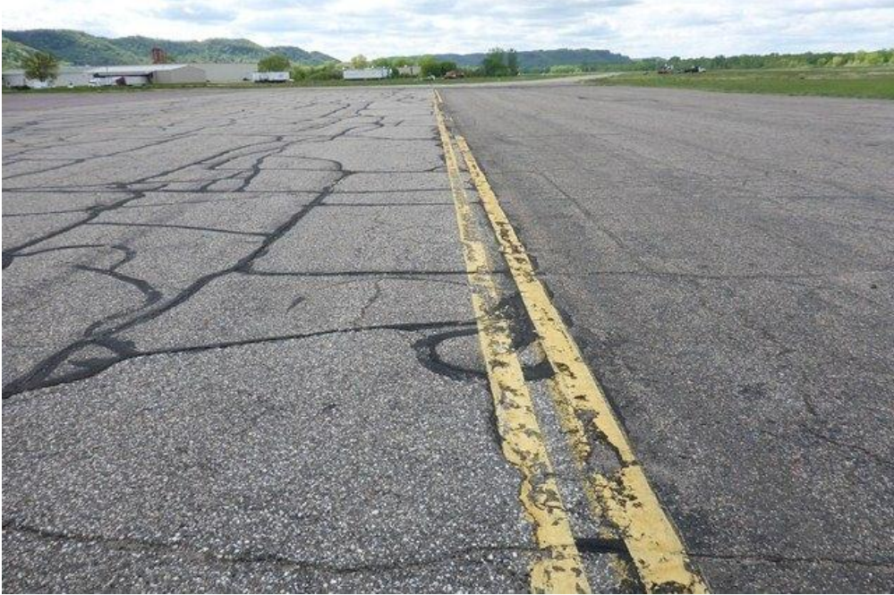
ONA APA 001 (Photo prior to 2015 Rehabilitation)
