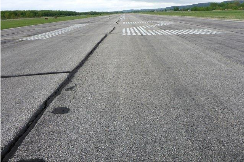
ONA RY1230 001 (Photo prior to 2015 Rehabilitation)
