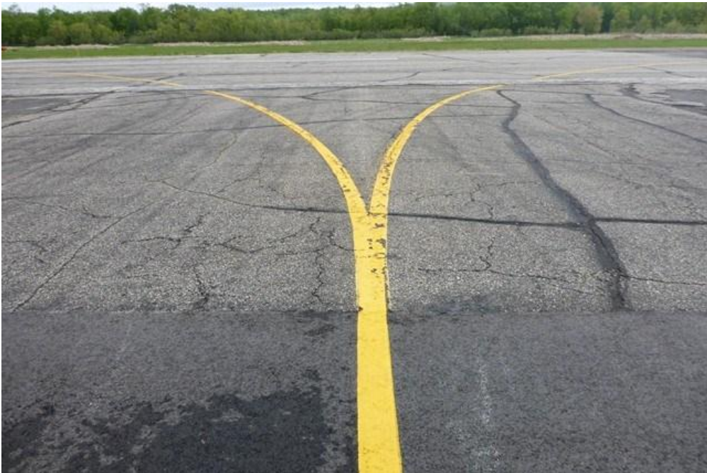
ONA CTA2 002 (Photo prior to 2015 Rehabilitation)
